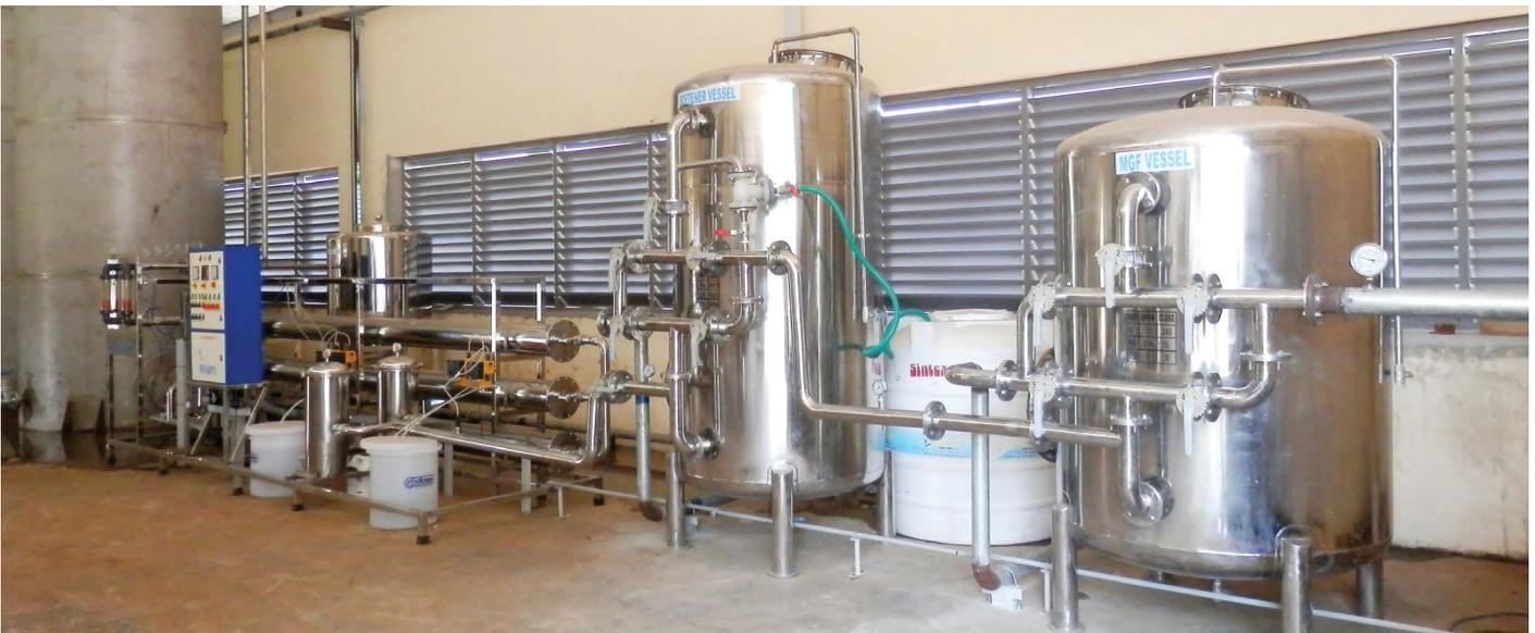
600 KLD Reverse Osmosis System for Boiler Feed
